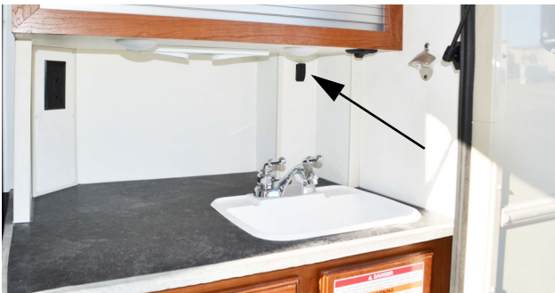
Tailgate Sink Drain Pump Switch (Located near exterior (tailgate) sink) -Typical View
